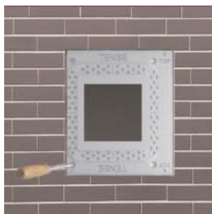
Screw the fixture on the wall by using 4 plugs and screws
